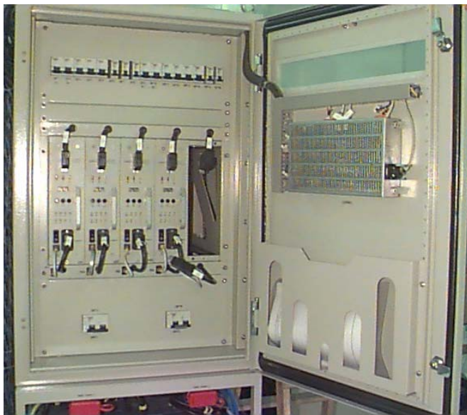
Figure 2. Basic power supply of -48\text{V}/250\text{ A} .
