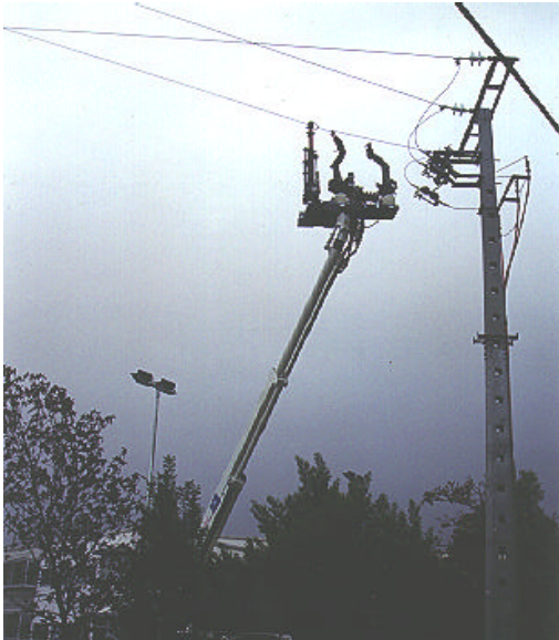
Figure 1. ROBTET system repairing a distribution line
